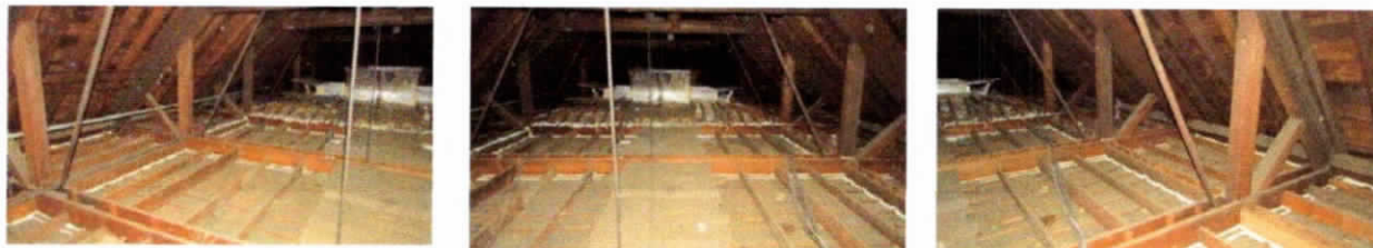
Photo 89 Attic prior to insulation
