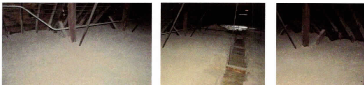
Photo 90 Attic following installation of cellulose insulation
