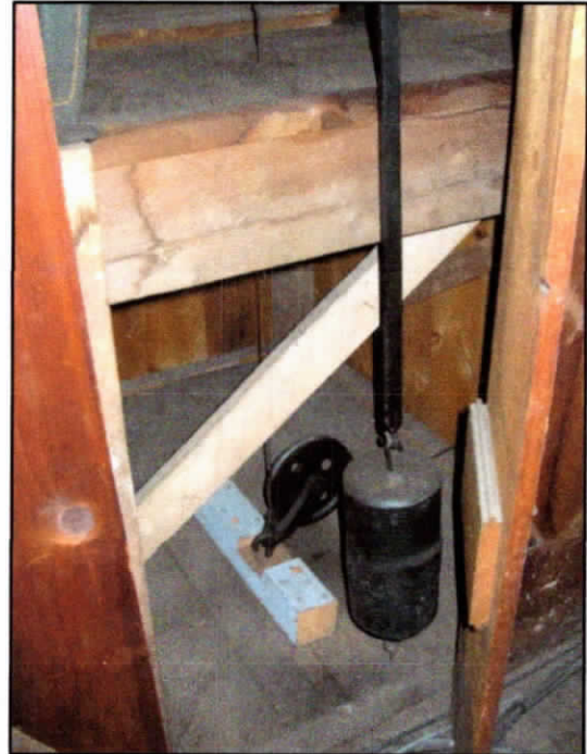
Photos 56 & 57 Clock movement and weight
