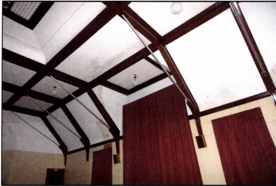
Photo 45 Detail of ceiling trusswork
